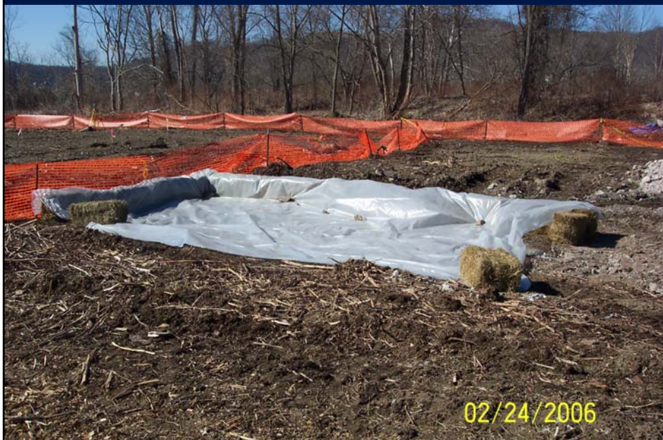
Hazardous waste containment area
