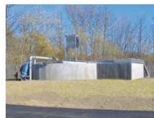
A view of Saco's new CSO treatment system.
