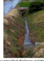
Baker provided drainage solutions to the City of Virginia Beach, VA, to address flooding problems that had existed for several years.
